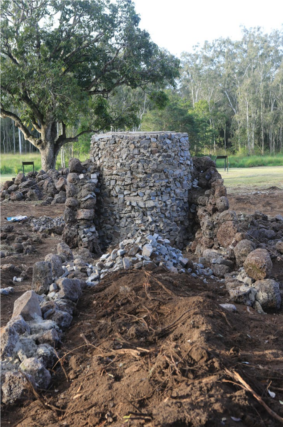
Figure 6.14 Oven completed with partially constructed ramp later filled with rock and soil, Atherton, Queensland. Photo: Gordon Grimwade 2016.
